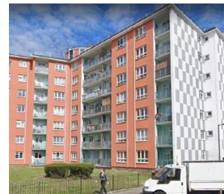
Southwark Park Estate
