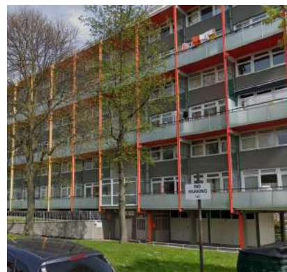
Dallas Road Estate, Lewisham
