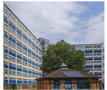
Wilmcote House, Plymouth City Council
