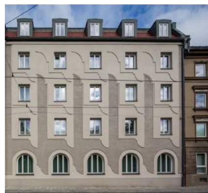
Munich. Housing block renovation.
