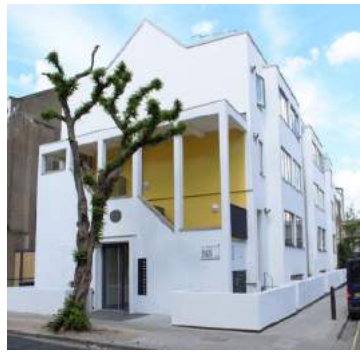
Artic Street, Housing Coop, Camden
